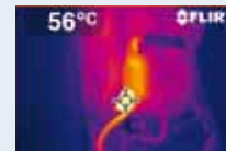
What a thermal imaging camera sees.
