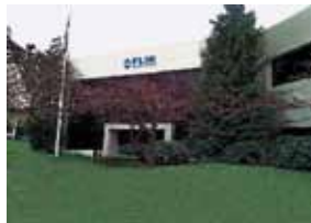
FLIR Systems, Portland
